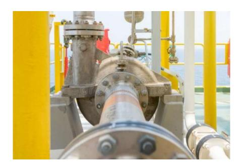
**2.1.1** *Pumps* (Components: seal, bearing, shaft, impeller, O-ring, casing, packing, coupling, nozzle)
